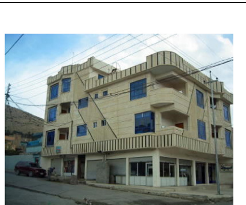
Sample intact building condition image
